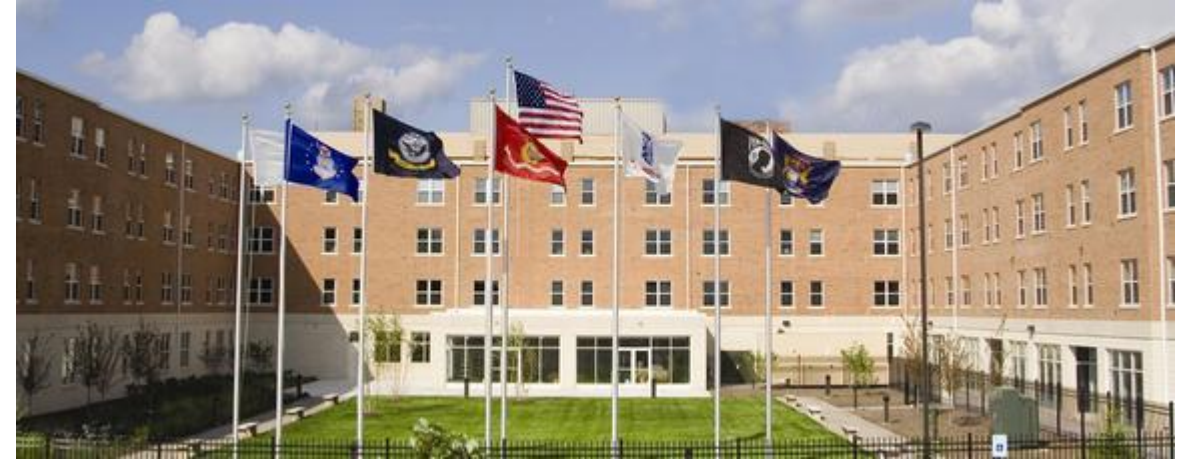
Piquette Square Apartments, Detroit, Michigan 150 Apartments for Homeless Veterans, Southwest Solutions
